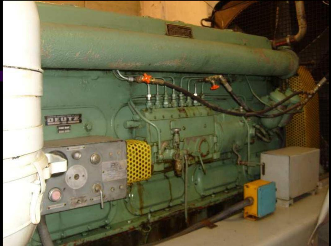
***Deutz 250 kW, 1500 rpm, diesel genset at DIME/SCL***
